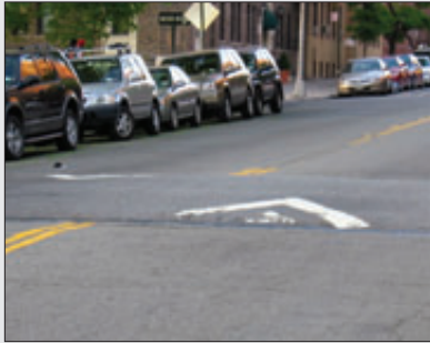
Figure 3.2.4 Speed table used to slow traffic in Inwood, Manhattan
