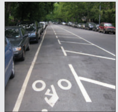
Figure 2.2.2 Buffered Class 2 bike lane in Park Slope, Brooklyn
