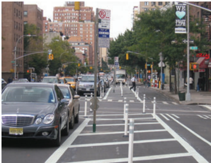
Figure 3.1.4 NYC DOT's 9th Ave. hybrid bike lane shifts parking to the outside of the bike lane.
