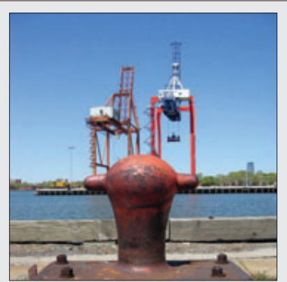
Figure 3.8.1 Maritime structures can serve as a railing or barrier
