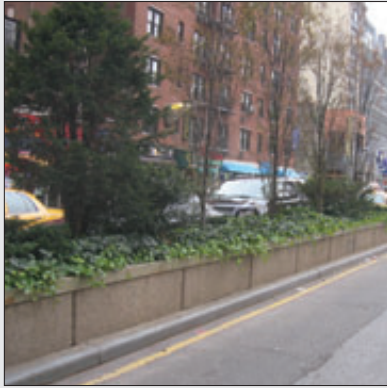
Figure 2.4.7 Side wall in street median of Union Square East in Manhattan
