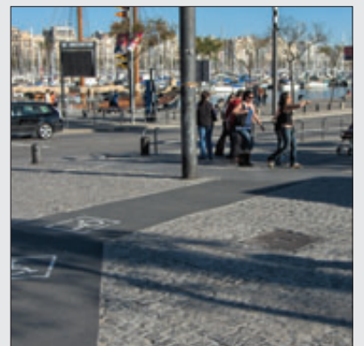
Figure 3.4.3 A paved strip to accommodate wheelchairs in Barcelona, Spain
