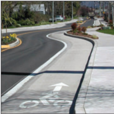
Figure 3.3.6 Three levels of grade separation
