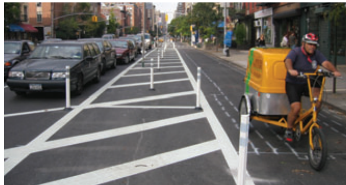
Figure 2.2.8 9th Ave Manhattan Hybrid lane painted buffer with bollards which will become planted buffers.
